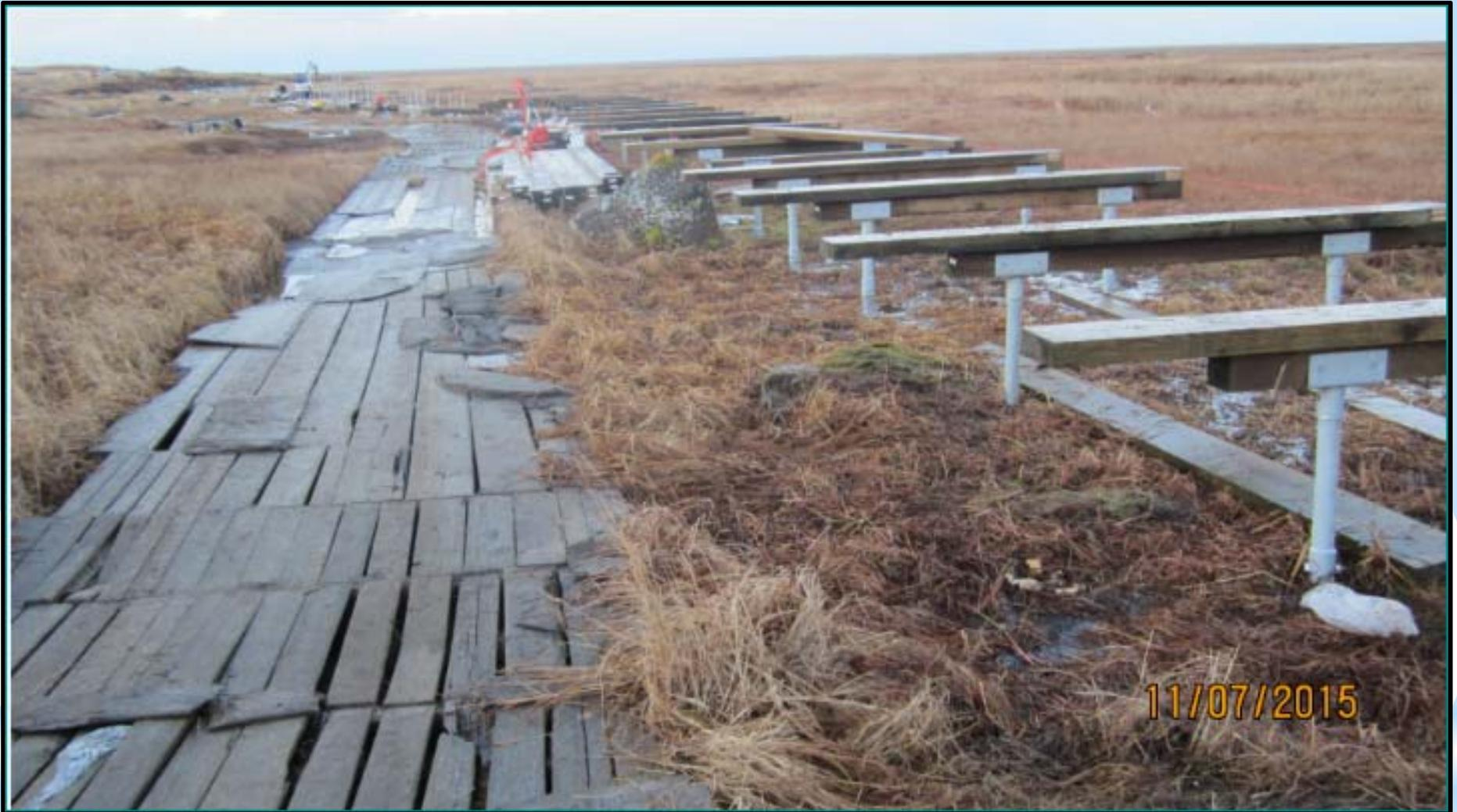
This shows the old boardwalk plus the new boardwalk that is under construction. We used the already-ordered 4x12 crossbeams as wide nailers on the 6x6 beams. This is about the same time we decided to make the deck 9 feet wide instead of 8'.
