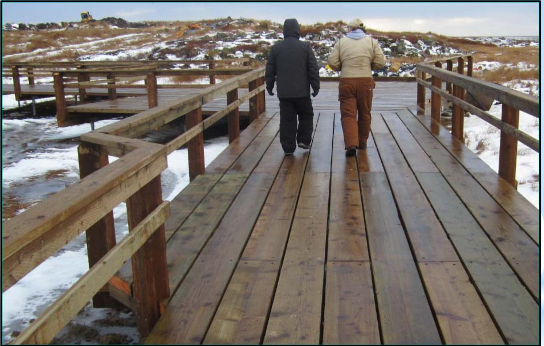
We made an 11-foot wide section just before the 28x35 platform to help our honey-bucket trailer have a little more turning room after the trailer is dumped.
