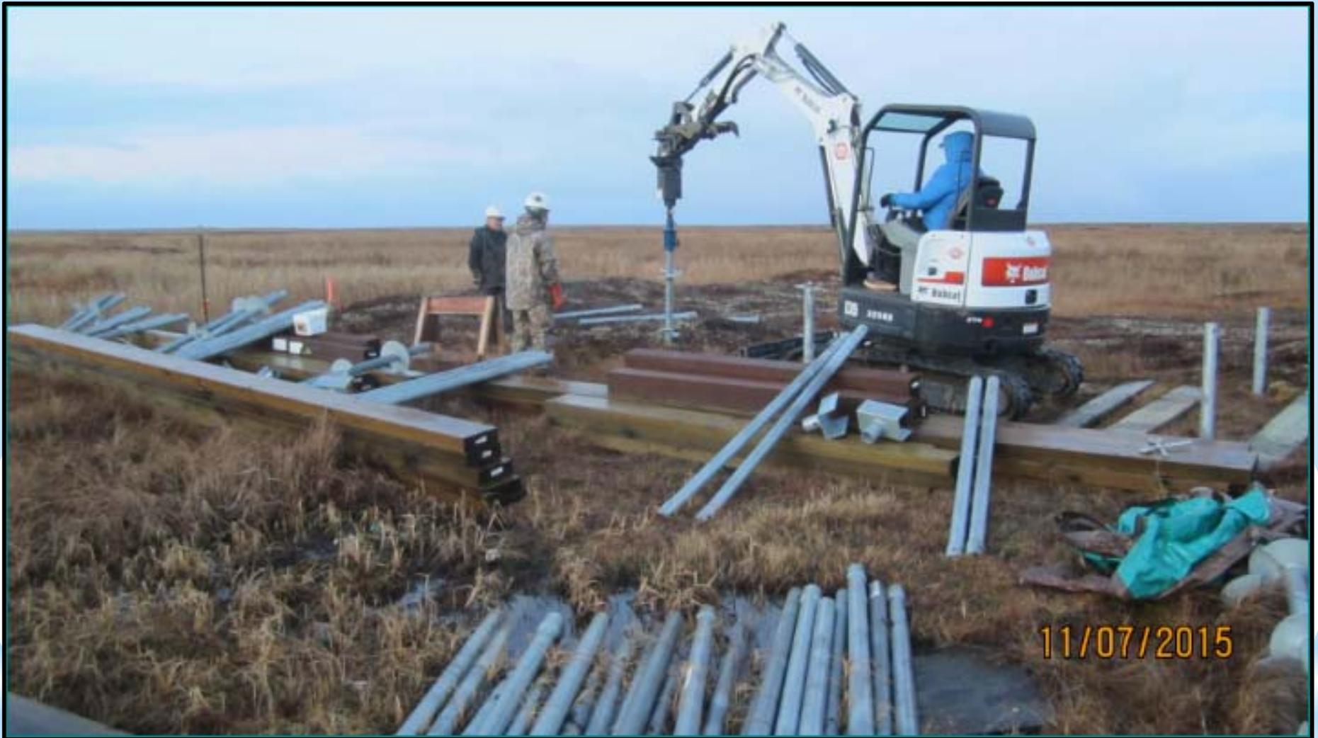
The hydraulic controls for the bucket's thumb on the City's Hitachi 300 excavator didn't work so would could not use our auger motor on the big excavator, yet. We decided to bring in a Bobcat mini-excavator on the last barge as a just-in-case.
