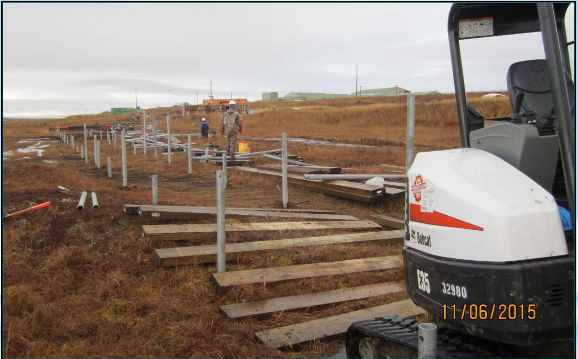
We used deck boards as mats to get across the soft ground. The softer the ground, the closer the boards were placed.
