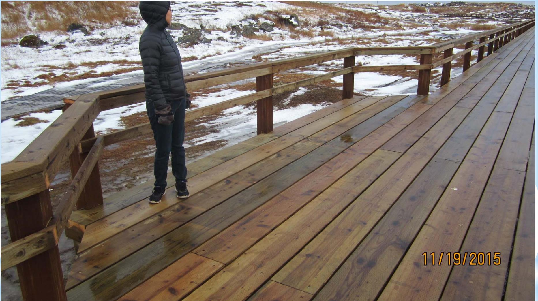
This is one of the two pullouts that we added to create a 13-foot wide section that will help the other ATVs when the honey-bucket trailer is on the boardwalk. This will help keep ATVs from having to back up several hundred feet in the fog.
