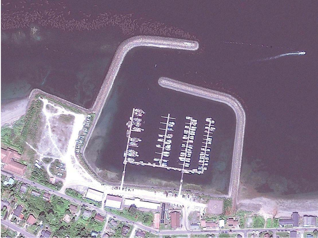
Aerial of New Harbor, 2009.
